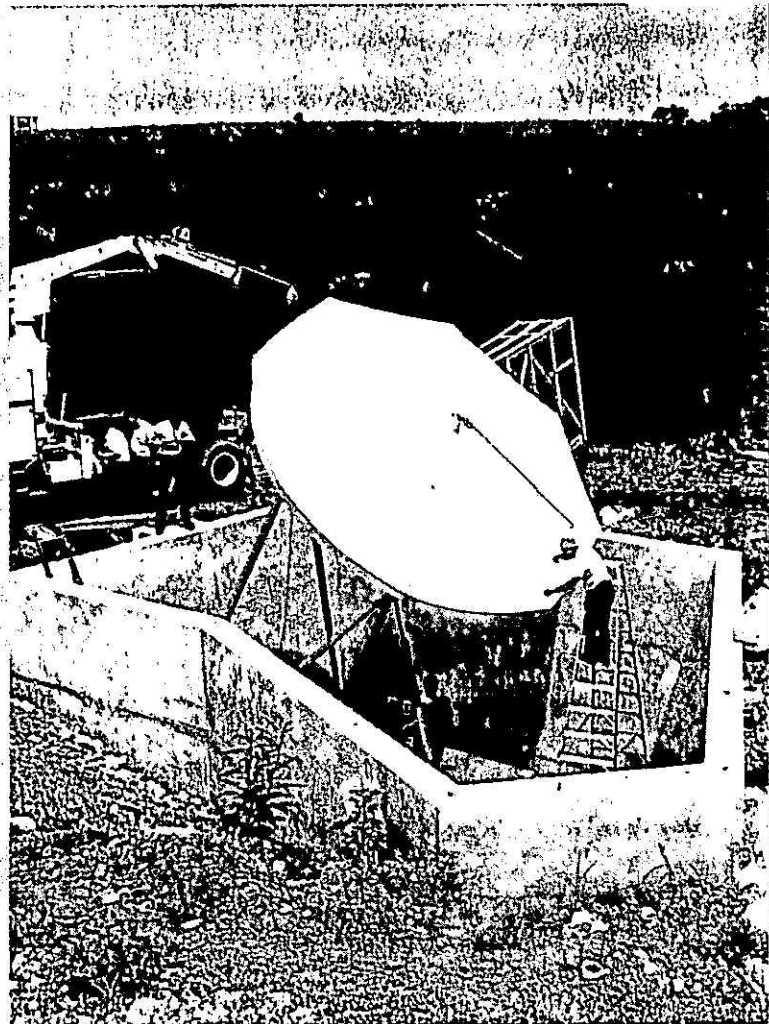
Showing one way to reduce interference from terrestrial signals, antenna at WEKU, Richmond, KY was installed in pit.
